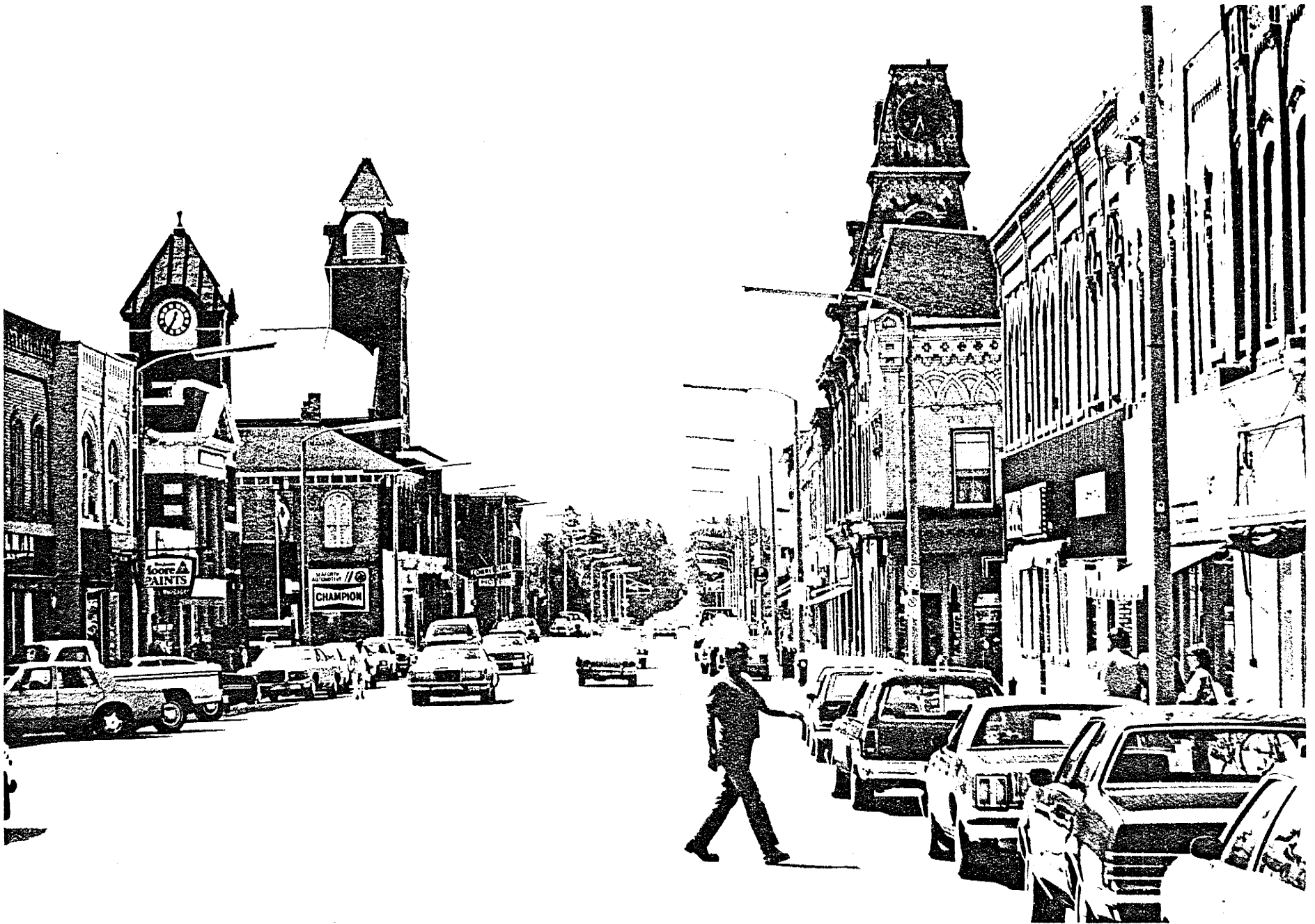
Main Street in Seaforth is one of the finest late nineteenth century streetscapes in Ontario. This picture shows well the variety of architectural composition consisting mainly of uniform commercial blocks with a marvellous roofscape of towers. There is that rare combination of order and spontaneity.
