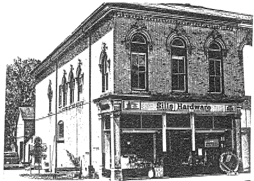
A full and profitable use of the entire building stock on Main Street is crucial for sound conservation.
